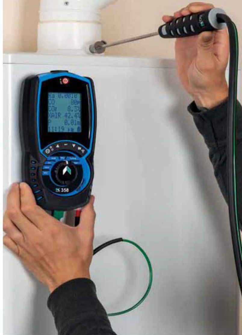
Flue Gas Analysis
