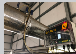
Gas Flow Monitoring
